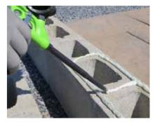
Structure Bond™ gun allows for a precise delivery with a single pull of the trigger.
