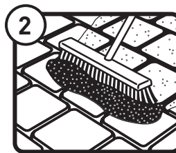
2 Using the street broom, fill joints completely. Spread sand over short distances .
